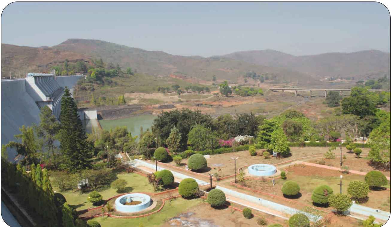
DAM OF UPPER KOLAB
