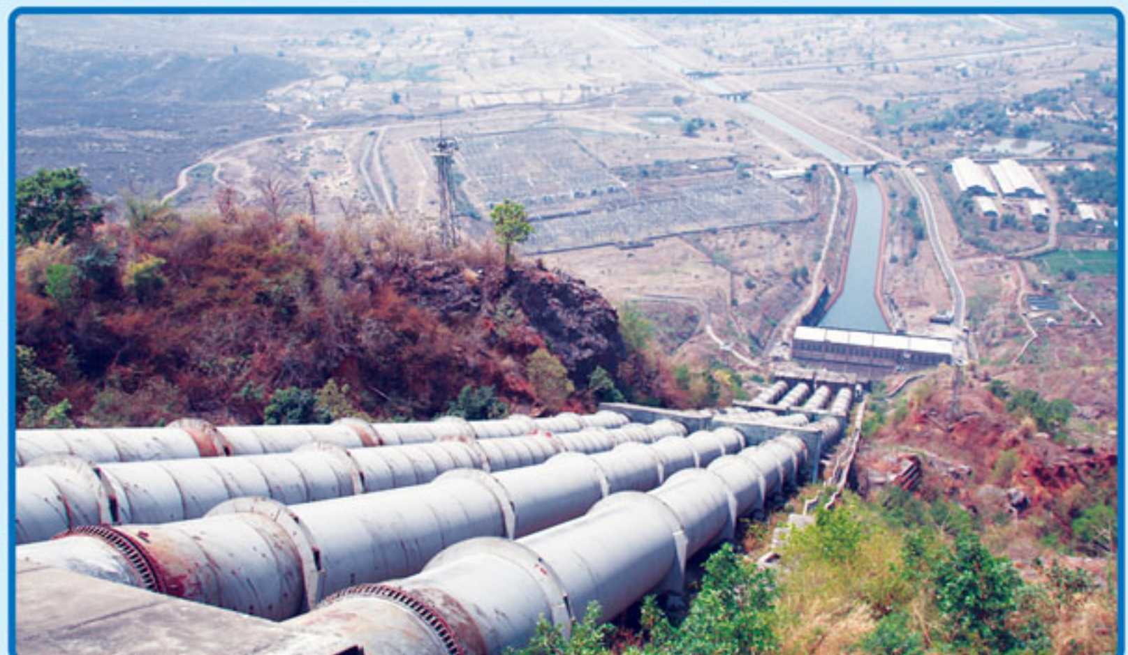
View from valve House Upper Indravati Power House.
