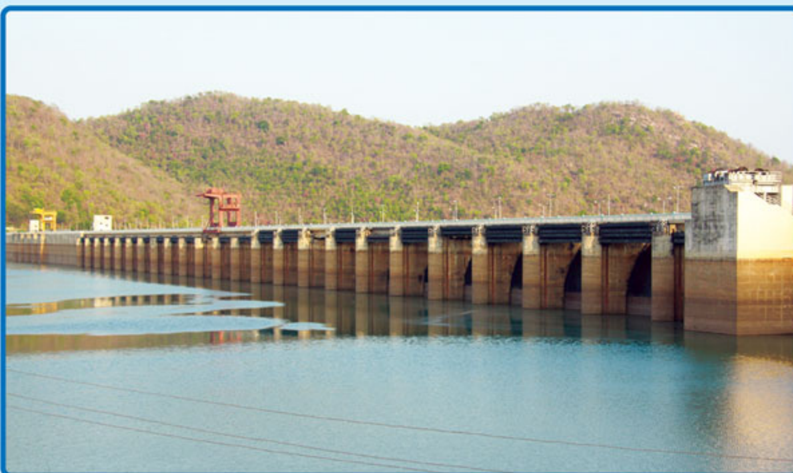
RHEP Dam, Rengali
